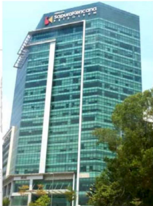
RENOVATION WORKS FOR KENCANA TOWER, KUALA LUMPUR
