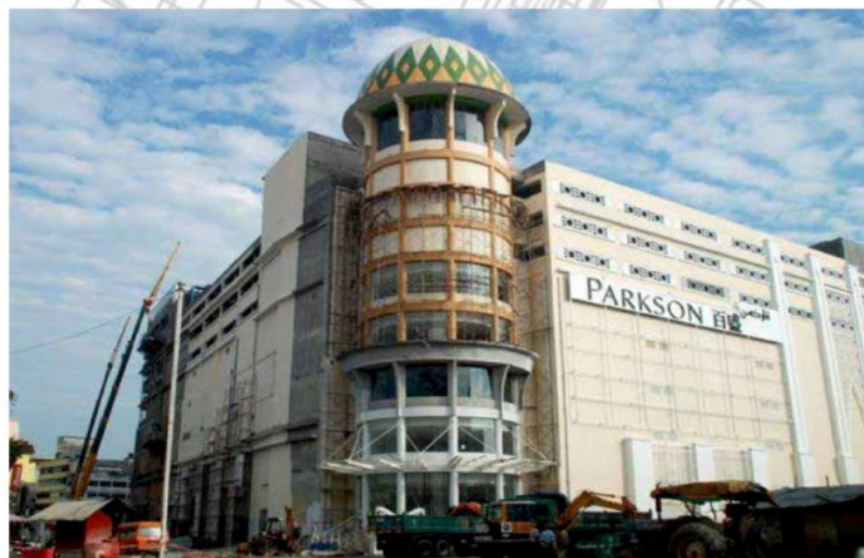
REFURBISHMENT WORKS FOR KELANTAN MALL, KOTA BAHRU
